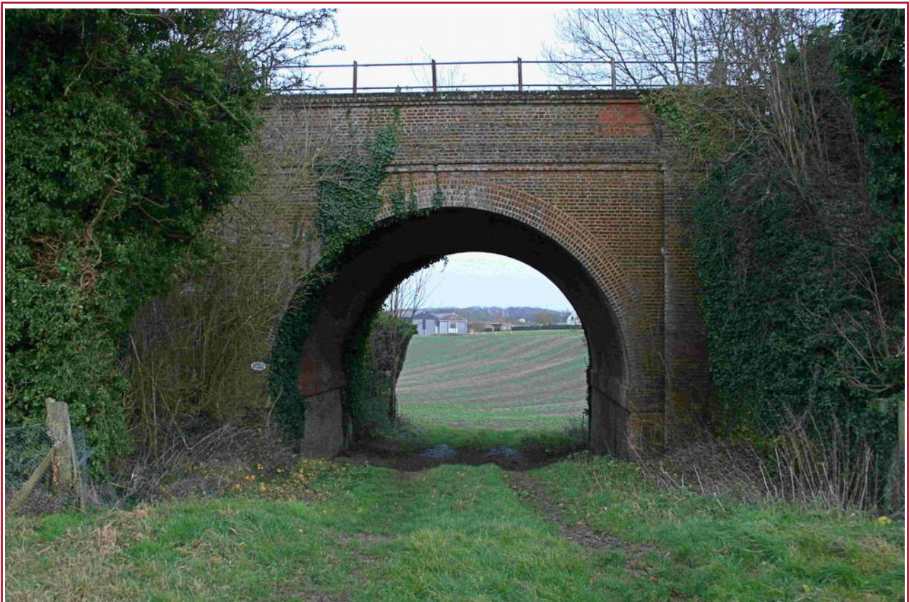
Illustration v: Railway bridge at B from north
